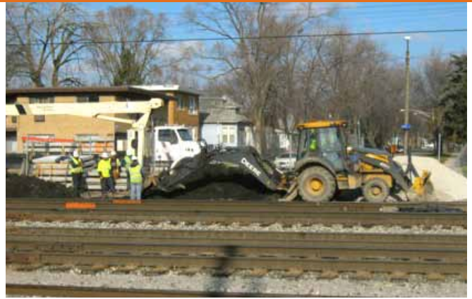
Signal installation at CP School Street progresses in December.
