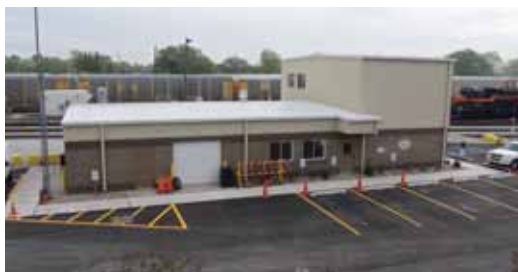
Crews completed the new Gibson Yard office earlier this spring.
