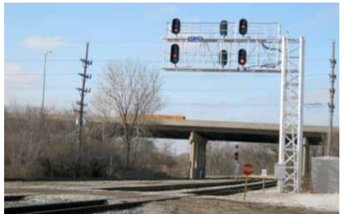
A westward view reveals progression of the B15 project in December.
