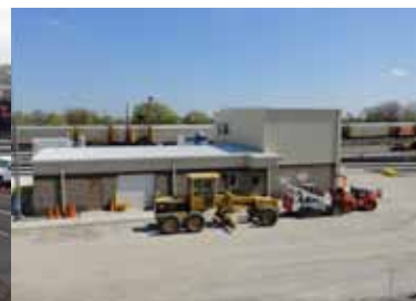
The adjacent parking lot is prepared for pavement April 12.
